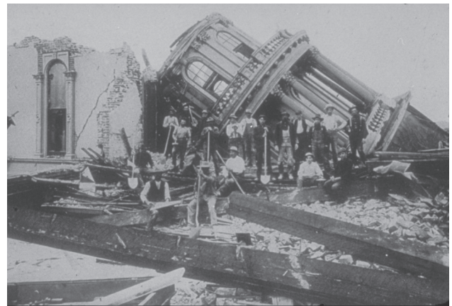
Collapse of City Hall at Santa Rosa, near San Francisco, 1906. [Image courtesy NOAA/NGDC, University of California-Berkeley.]
