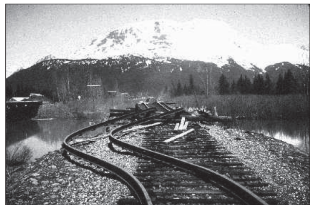
Turnagain Arm, railroad torn during 1964 earthquake. [USGS photo by Joseph K. McGregor and Carl Abston.]
